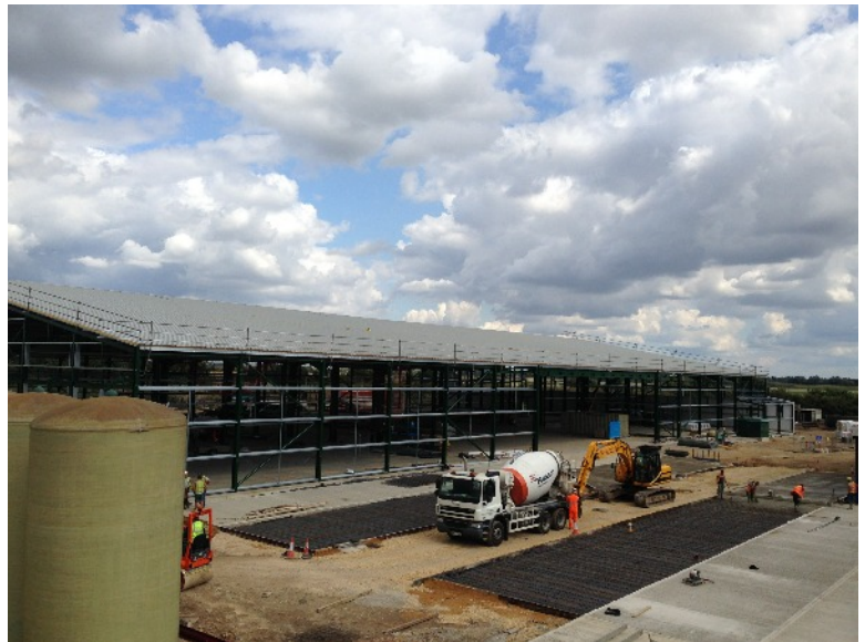
The site during construction
